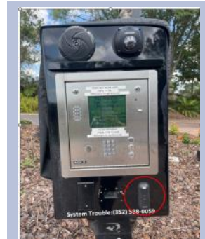
Front Gate Kiosk
